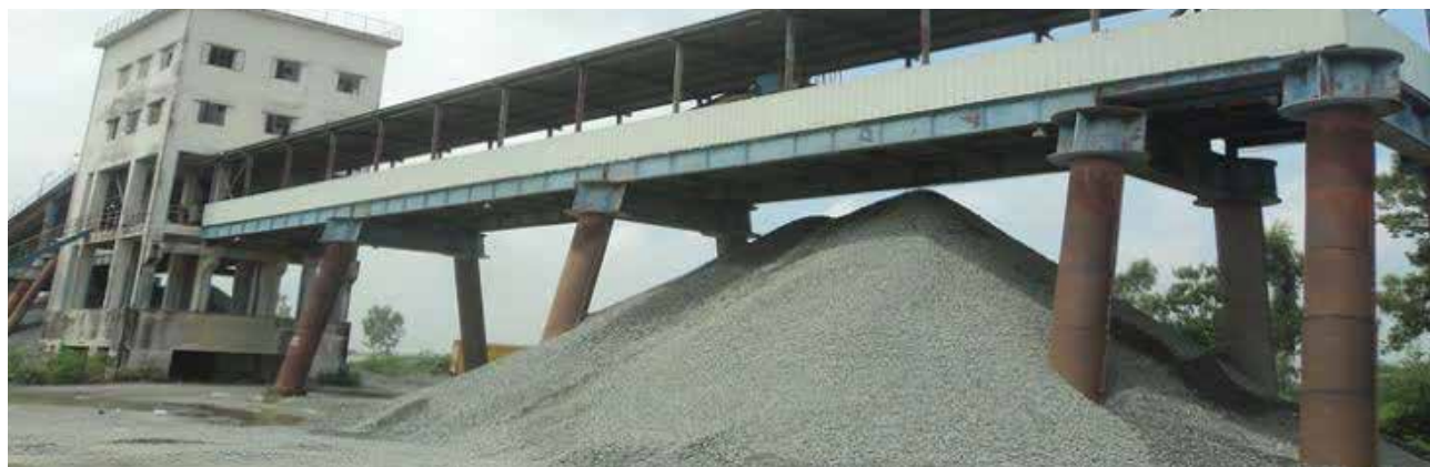
► Granite Rock Batching Yard
