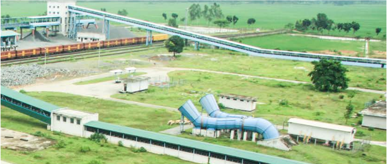
Loading and transportation system of Granite Rock
